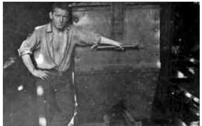
Tom Moran filling the fires in no. 3 house.
