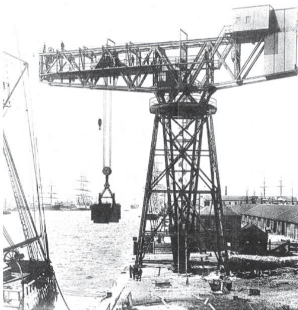
Testing the 100 ton crane, circa 1905.
