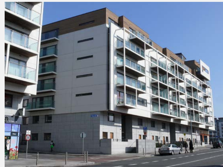
136/137 Gallery Quay apartments under construction in 2003 and completed in 2009 (Astrid Wonneberger).
