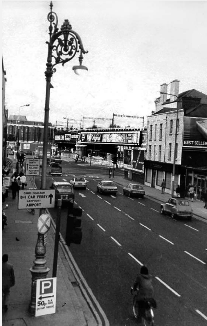
153 The new Tara Street Bridge and Loipline Bridge in 1986 (St Andrew's Archive).
