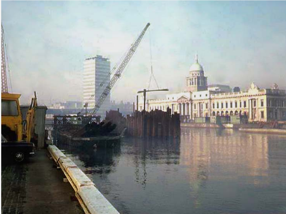
148 The construction of the Matt Talbot Memorial Bridge in 1976-1978 (St Andrew's Archive).
