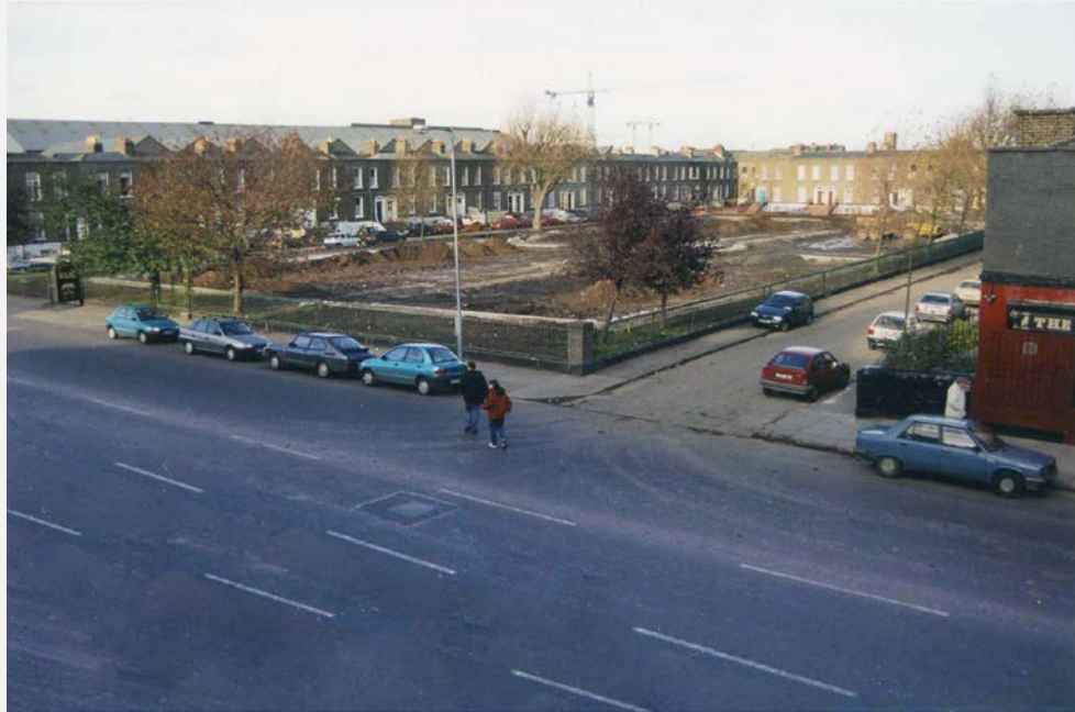
159 Pearse Square undergoing refurbishment in 1996 (St Andrew's Archive).
