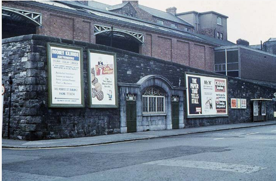
124 The men's toilets on Pearse Street in the 1970s (St Andrew's Archive).
