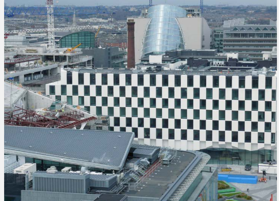
37 Aerial View of the Gallery Quay development taken from the Altro Vetro building on MacMahon Bridge in 2009 (Astrid Wonneberger).
