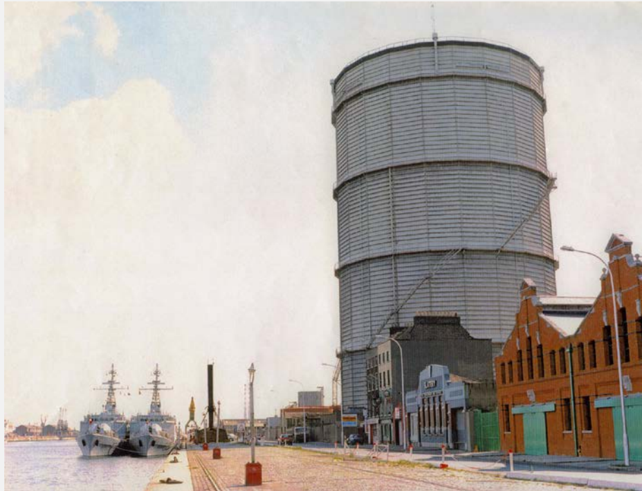
11 The Gasometer, located on the Gas Company site at the junction of Sir John Rogerson's Quay and Cardiff Lane was erected in 1934. It became a very well known landmark in the city before it was dismantled in 1993 to make way for the development of the "Old Gas Company" site (St Andrew's Archive, 1980s).
