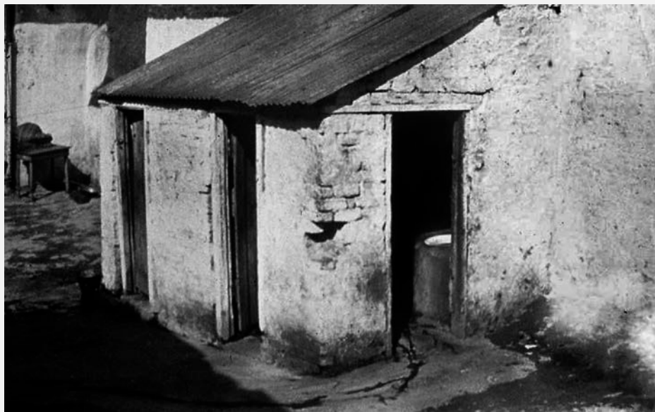
120 Toilet in the back yard (ca. 1950s) (St Andrew's Archive).
