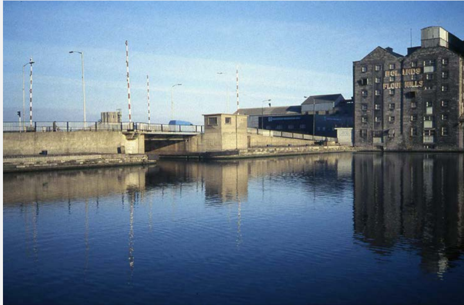
161 MacMahon Bridge and Boland's Mills in the late 1980s (St Andrew's Archive).
