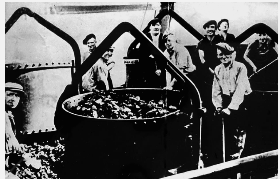
51 Val Harris and men working coal in the late 1940s (St Andrew's Archive).
