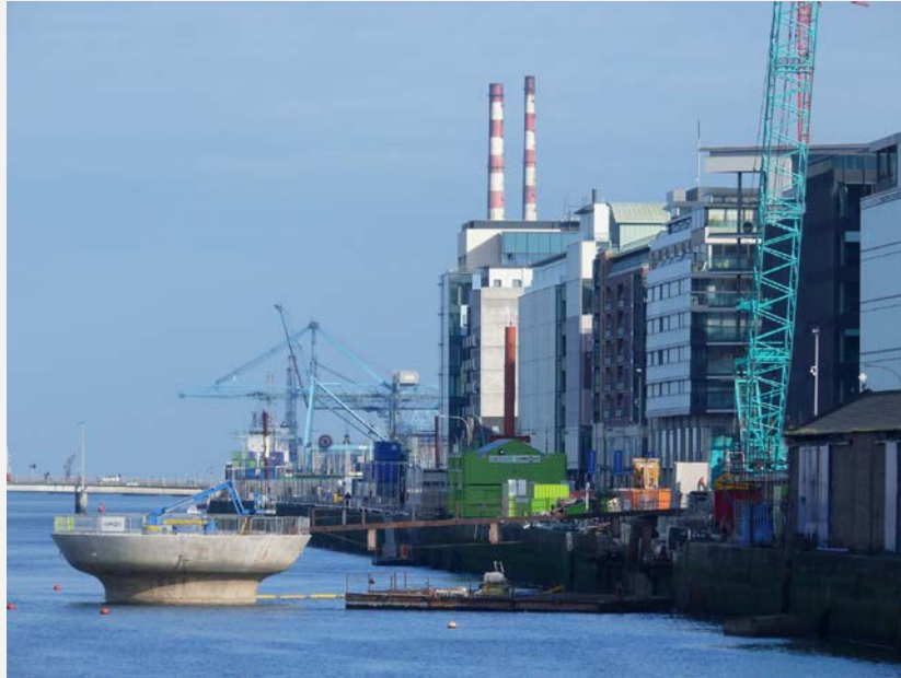
150 The construction of the new Samuel Beckett Bridge (aka Macken Street Bridge) in 2009 (Astrid Wonneberger).
