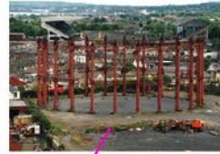
Gasometer Barrow Street
