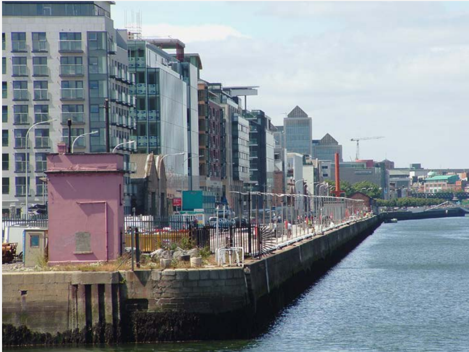
9 The Hailing Station on Sir John Rogerson's Quay shortly before its demolition in 2007 (Astrid Wonneberger).
