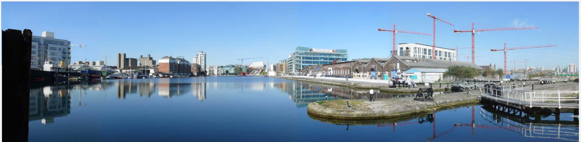
176/177 Panoramic view of the locks, Grand Canal Dock Basin and Britain Quay in the 1980s (St Andrew's Archive) and in 2009 (Astrid Wonneberger).
