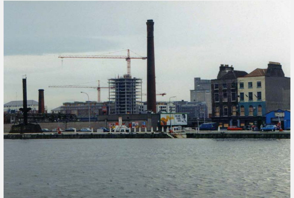
24 The Gas Company site after the demolition of the Gasometer in 1993, viewed from the North Wall Quay in the late 1990s. Note the construction of the Millennium Tower at the Grand Canal Basin (Richie Kelly).
