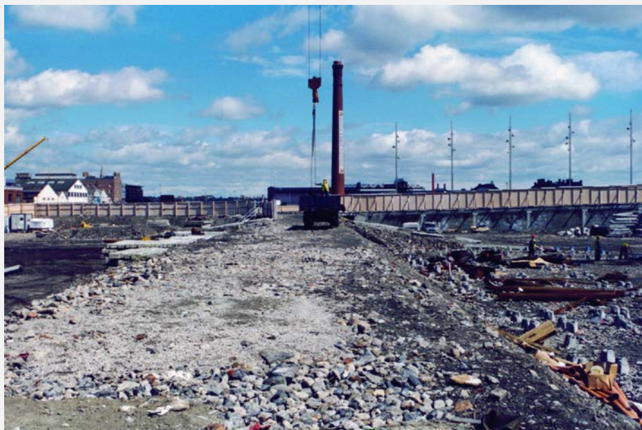
18 Decontaminating the Gas Company Site in 2003 (Astrid Wonneberger).
